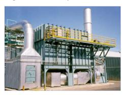
Although thermal oxidation is recognized as the best solution to destroy VOCs, the challenge is to minimize fuel and operating costs of the process.
