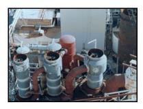
Pre-evaporation systems utilize low-level waste heat (where available) to evaporate weak liquor prior to the main evaporator train. Aside from using waste heat, one of the main advantages of a pre-evaporation system is condensate segregation. The ideal scenario for a mill with a pre-evaporation system is to use separate liquor storage tanks for the virgin weak liquor and liquor that has been through the pre-evaporator.
