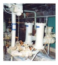
Strainers and filters are used to remove suspended contaminants from an aqueous, organic or gaseous stream in order to produce a higher purity product.
