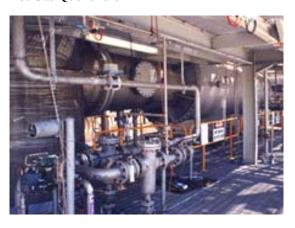
Excessive heat entrained in gas streams can be effectively removed by direct injection of water or other liquids into the gas stream, utilizing evaporative cooling. Our quench vessels are designed to introduce fine aerosol sprays at critical positions on the vessel to achieve the most efficient absorption of the liquid without carry-over.
